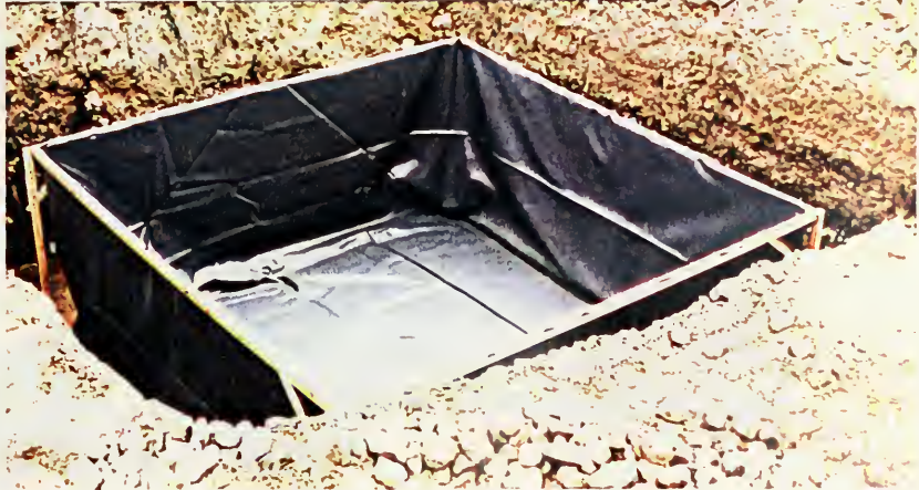
A7: FRAME AND LINER IN POSITION
